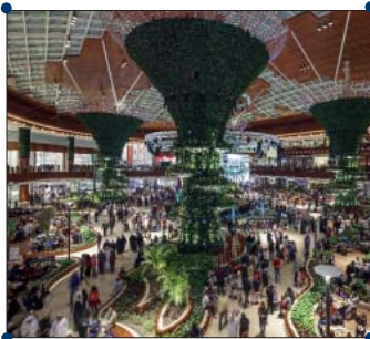
Mall of Qatar Al Rayyan, Qatar Developer: Urbacon Trading and Contracting Architect: Chapman Taylor
