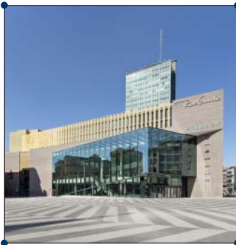
Rive Gauche Charleroi, Belgium Developer: Saint-Lambert promotion c/o Iret Development Architect: DDS+ Other: MS-A, Air Design, D Interieur, Valens-Duchène, Franki, Kone, Druart
